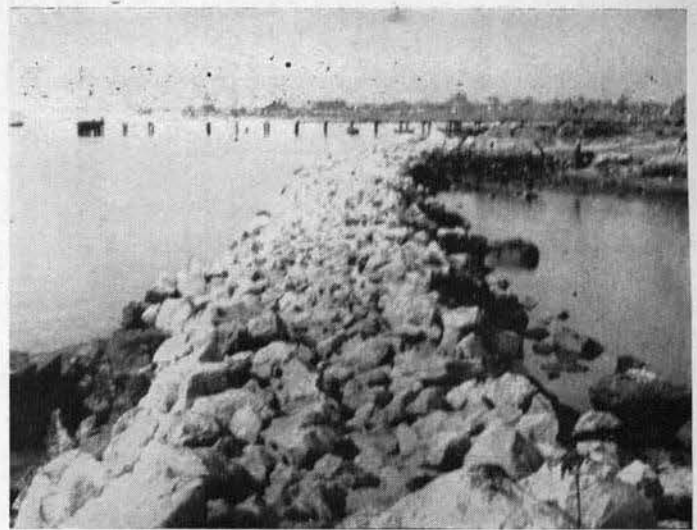
Arranque. Escollera Norte.—Tampico, Tamps.
